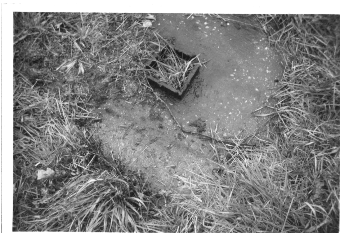
This looks like an old aerial tower support that has been cut down for scrap. Note the date "1946" carved into the concrete by the builder!
