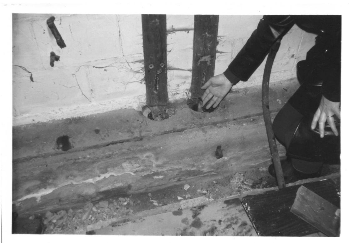
This is one of the coaxial feeder cables from the aerials.
