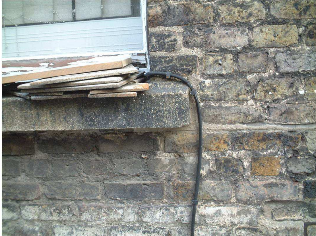
Figure 62: 3Mbps Ethernet cabling at Dept. Computer Science, TCD Photo courtesy Mike Nowlan
