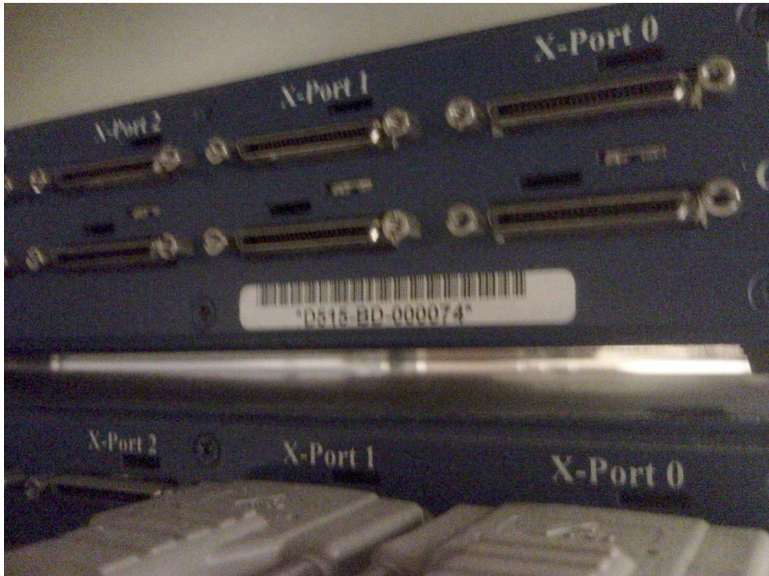
Figure 8: CAGcluster0 SCI switches after removal, rear closeup
