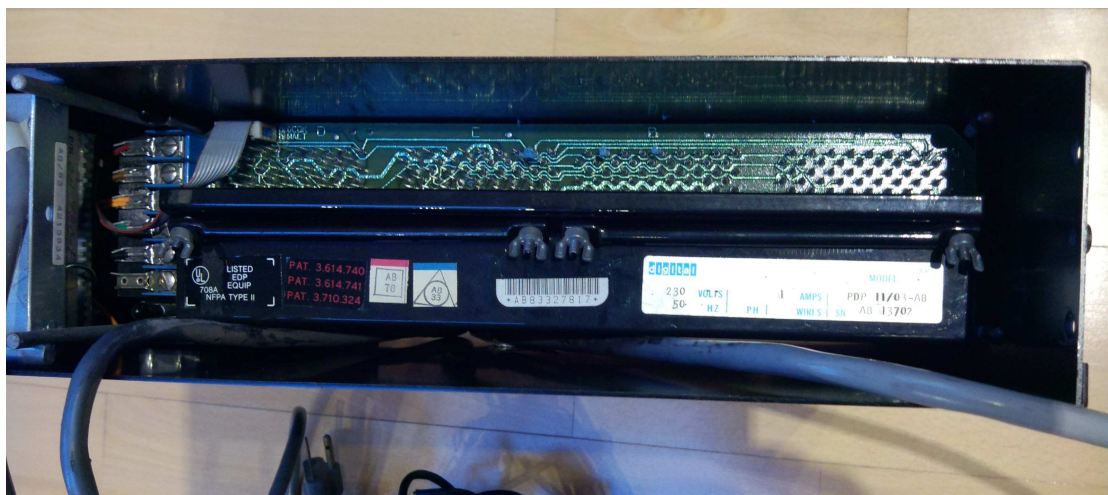
Figure 16: DEC VAX 11/780 Console Processor Qbus backplane closeup
